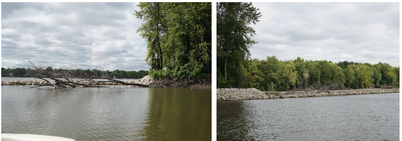
Figure 15: Anchored Felled Tree at Beaver Island HREP (USACE photos).
