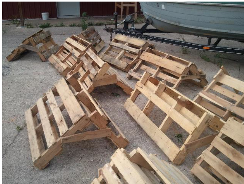
Figure 14: Fish Habitat Pallet Structures (USACE photo).
